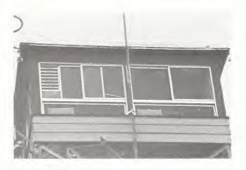
Figure 222. The cab of Horsethief lookout, with new siding and aluminum sliding windows.
